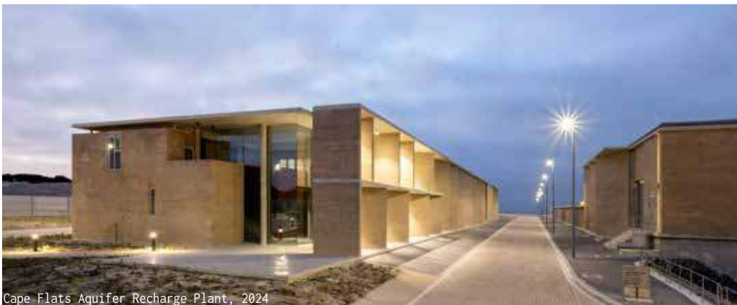
Cape Flats Aquifer Recharge Plant, 2024
